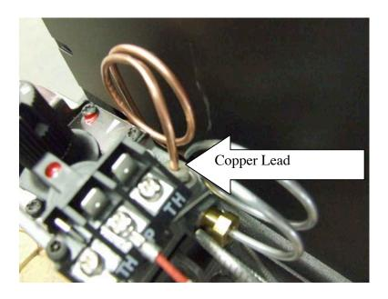
5. From underneath the stove, use wire cutters to cut the copper colored lead to the thermocouple as close to the fastening nut as possible. DO NOT CUT THE ALUMINUM GAS LINE!
